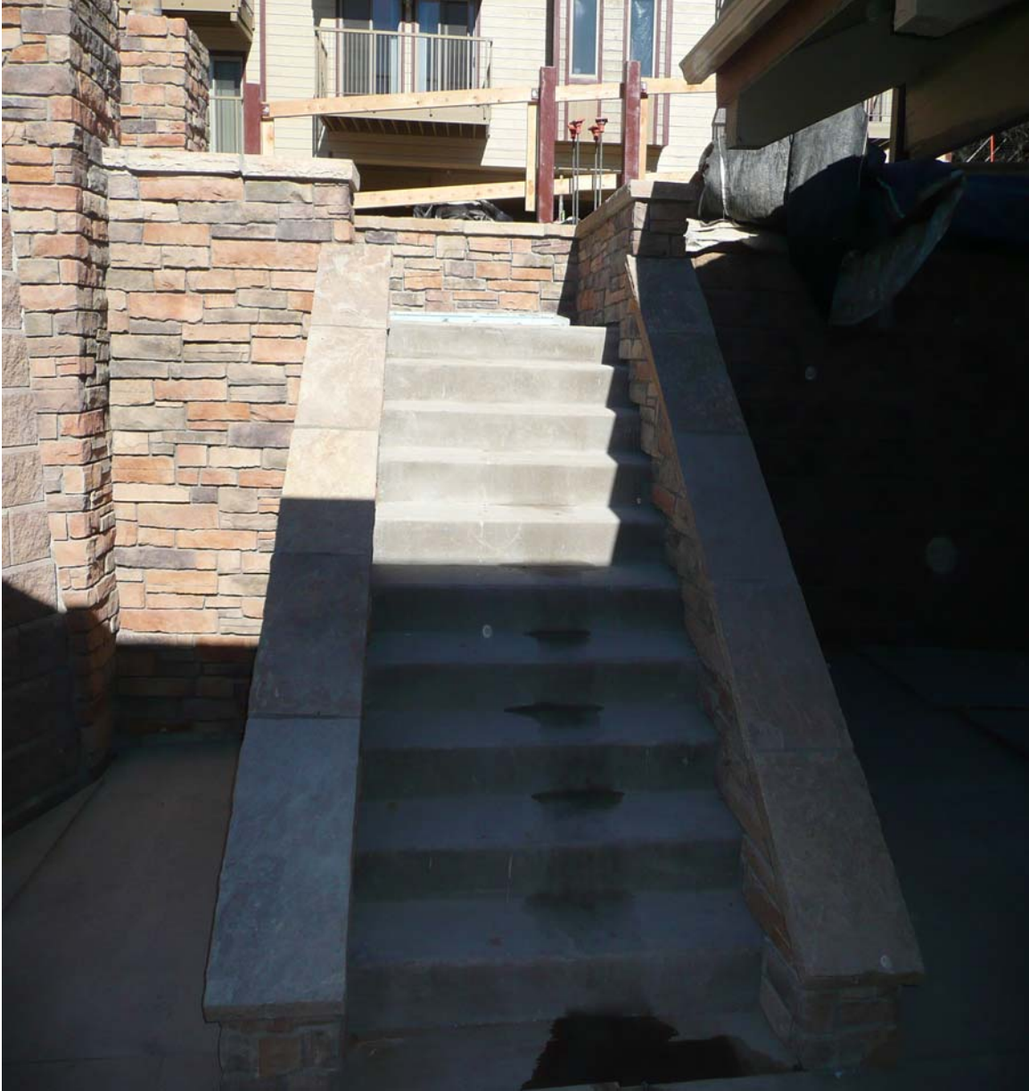
Steps Leading Down to Building A's Office (View 2/2)
