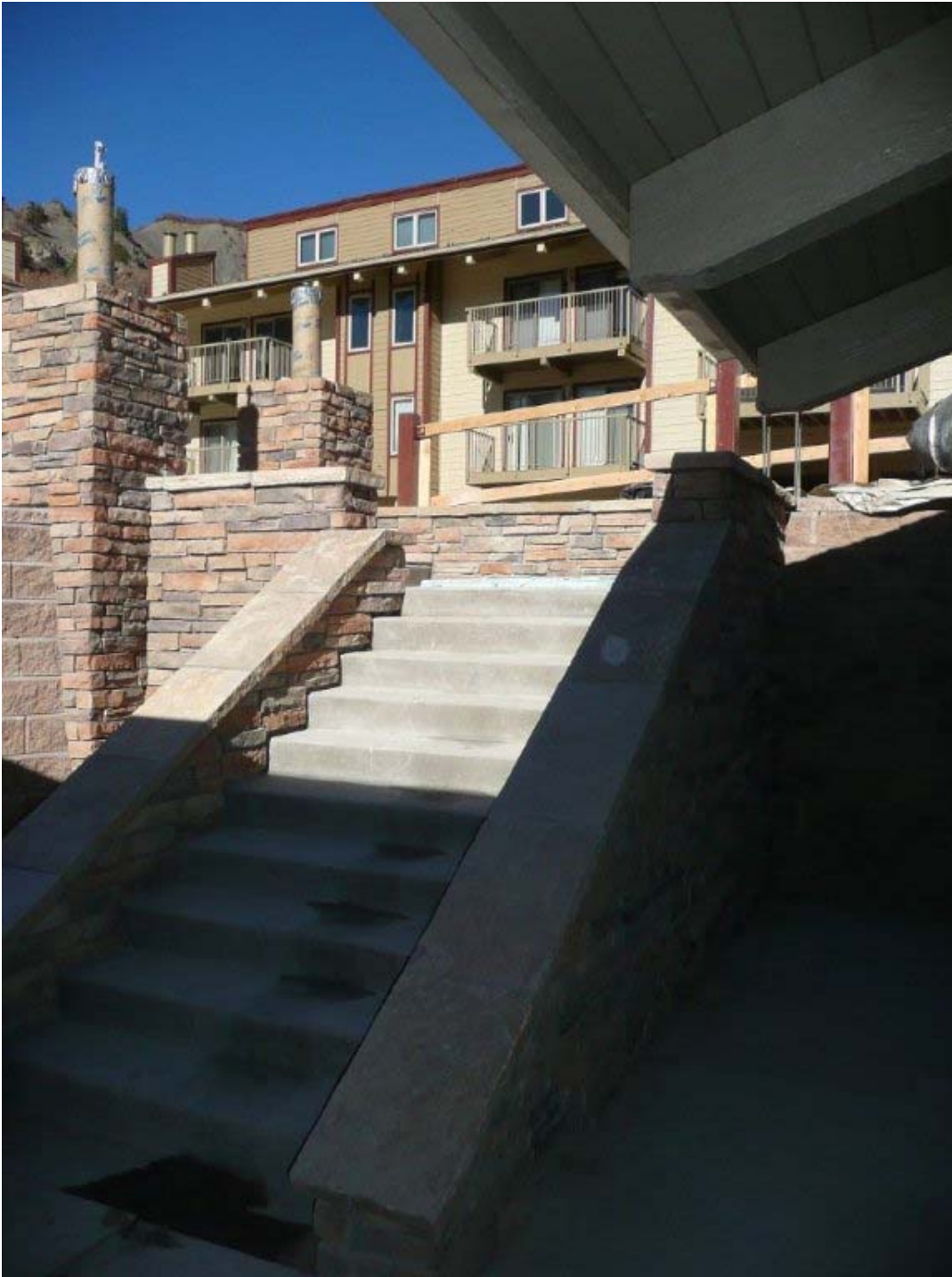
Steps Leading Down to Building A's Office (View 1/2)
