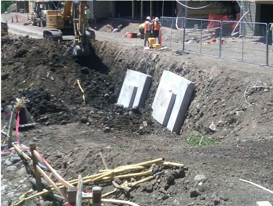
Final picture shows a shoring block being positioned into place.
