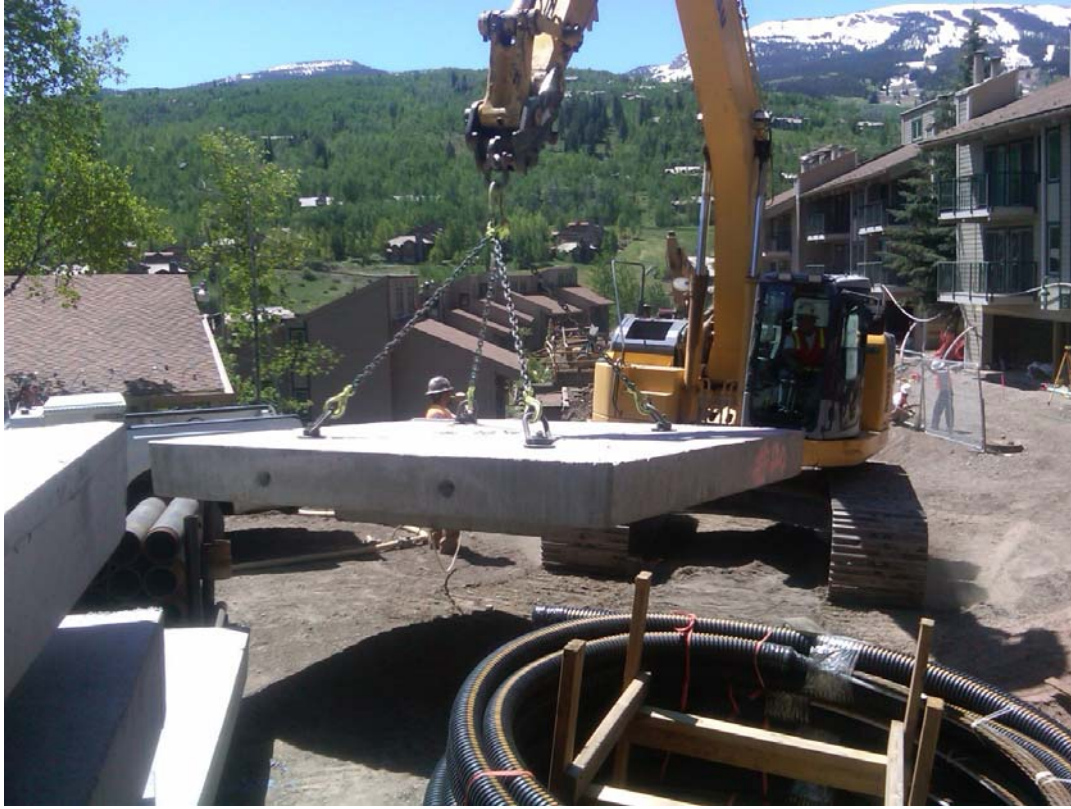
Final picture shows a shoring block being positioned into place.
