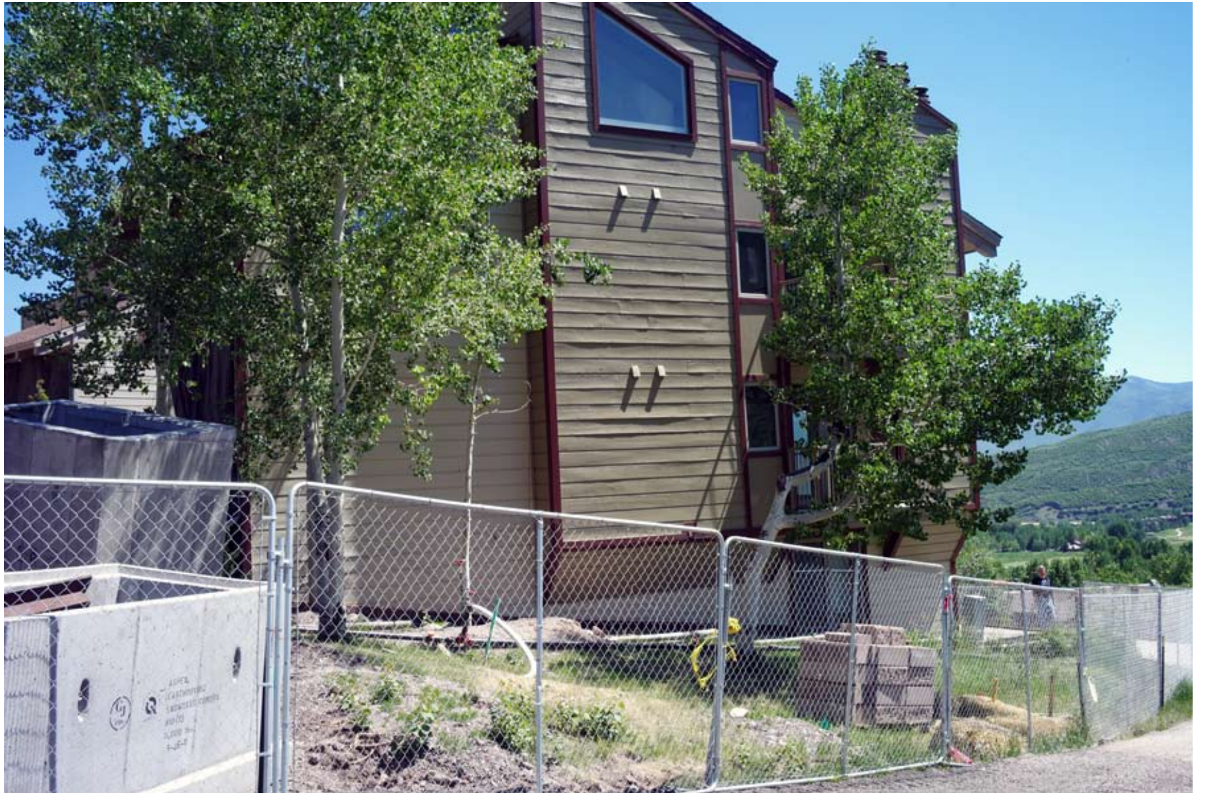
3 Entryway Building L side Showing Area Where Sign Was Removed
