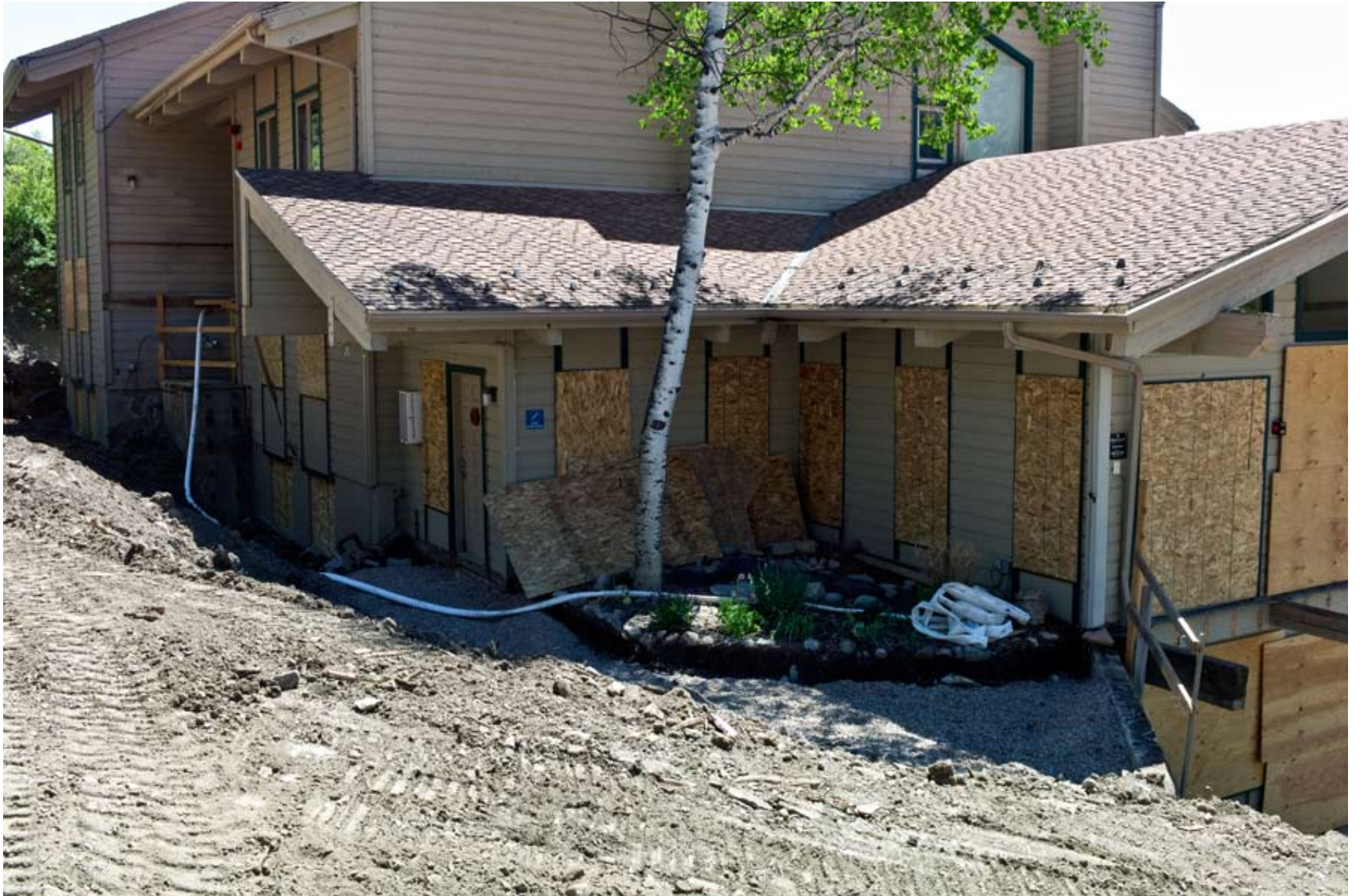
5 Building A Entry to Office Pool Conference June 29 2011 1
