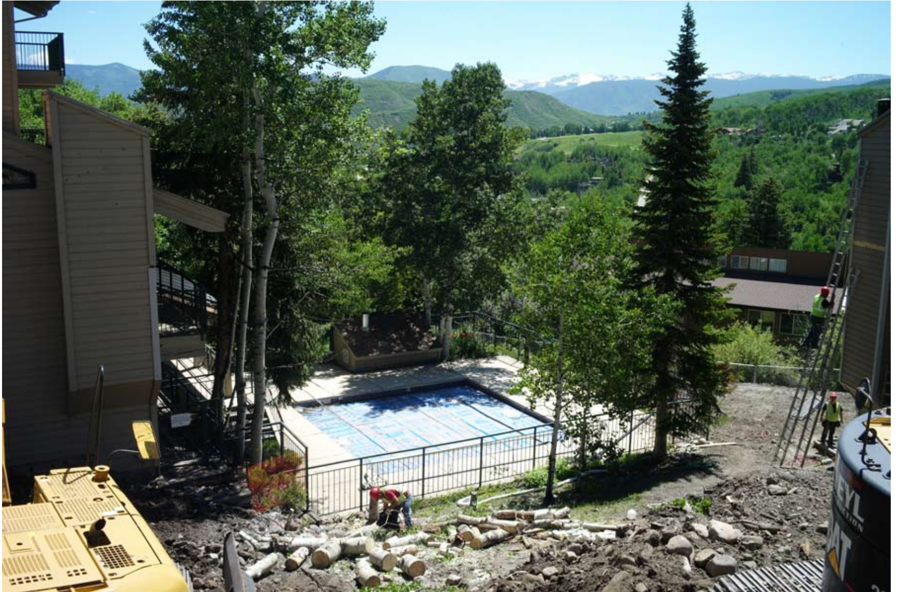
6 Pool View from Roadway Adjacent to Building A 1
