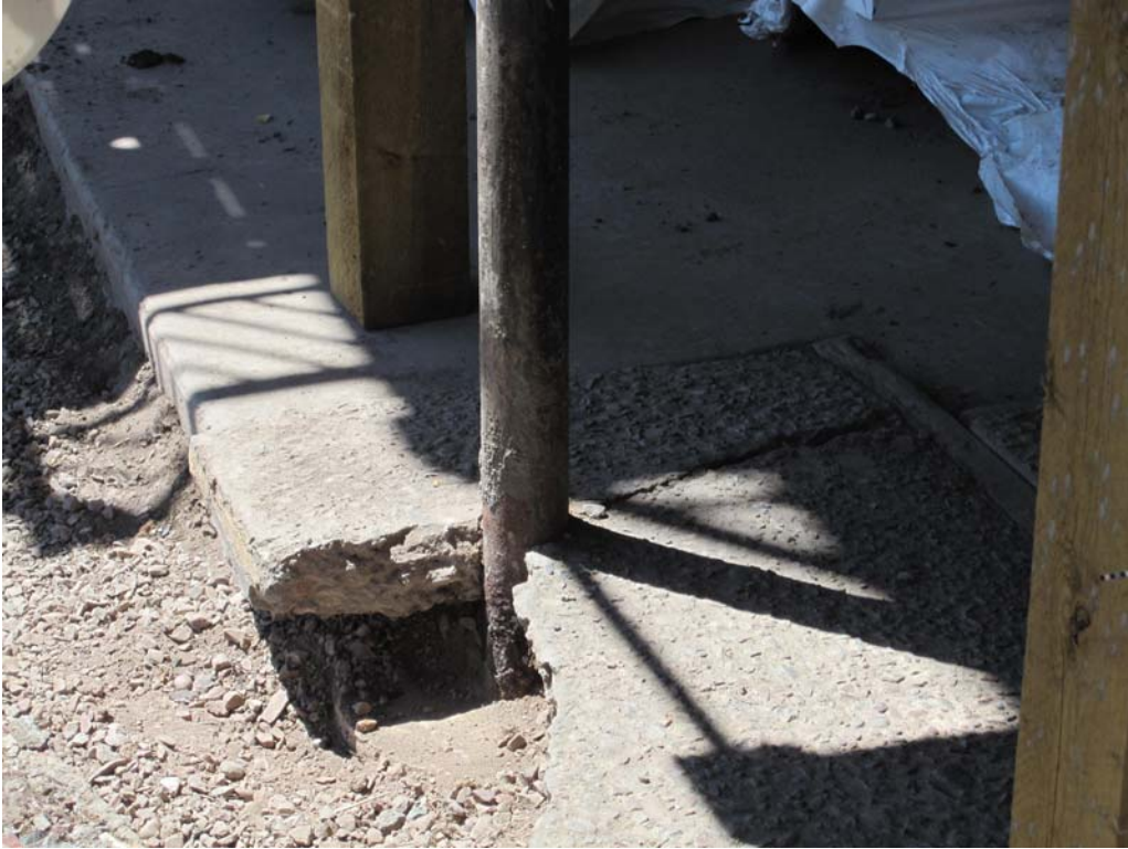
Above : The Problem – support poles that are off-plumb and corroded below the surface. Below: Bill Perry, Hank Hayes, George Falk, and John Meckling talk over possible solutions.
