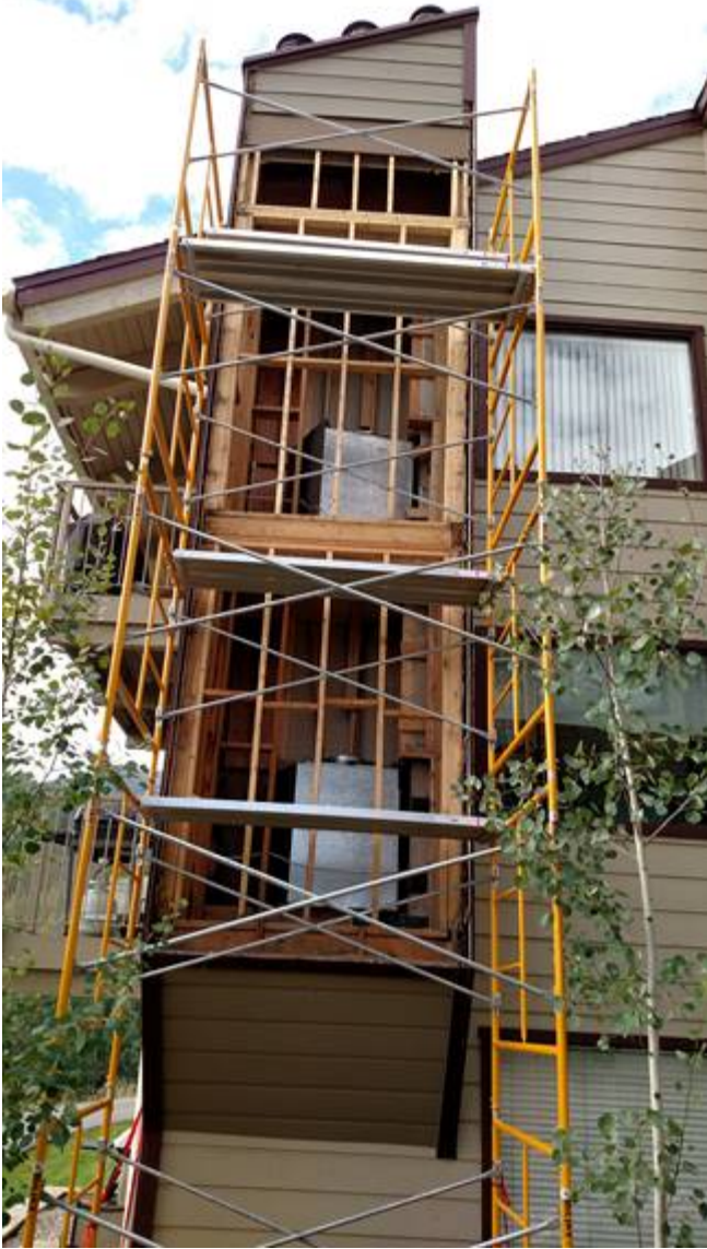
Figure 3 - North chase Bldg K (fireboxes are pulled back but awaiting hand-crane to remove from the chase)
