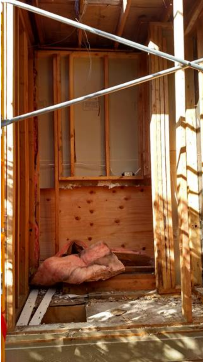
Figure 9 - Inside of a chase
