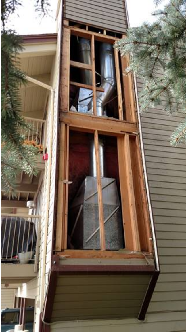
Figure 2 - North chase Bldg D
