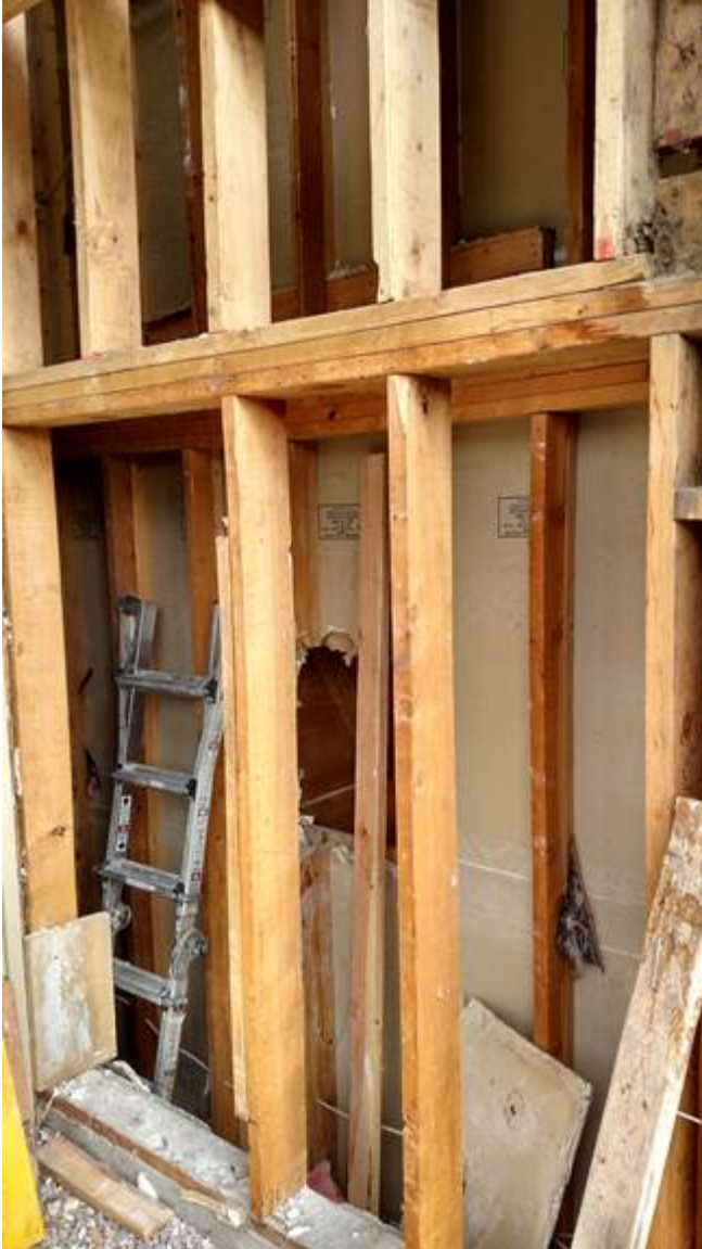
Figure 4 - Clearing old materials from middle chase Bldgs J/K
