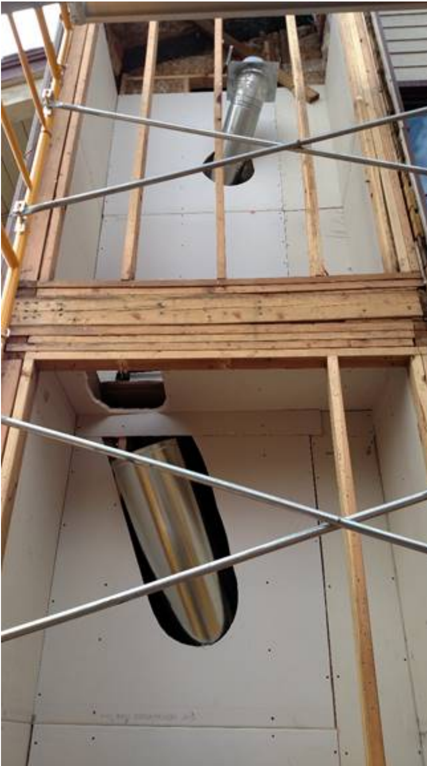
Figure 2 - Drywall and flues Building B
