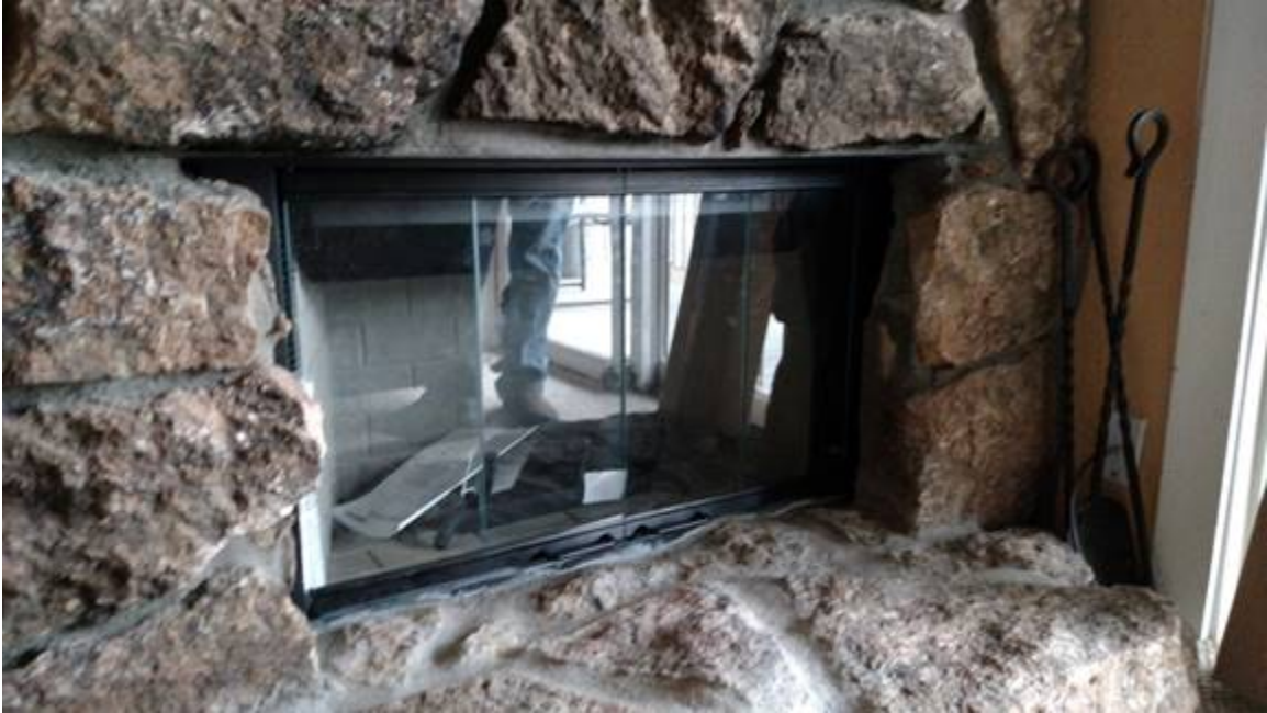
Figure 2 - this is one of the units that needed adjustments to the existing stone... came out great.
